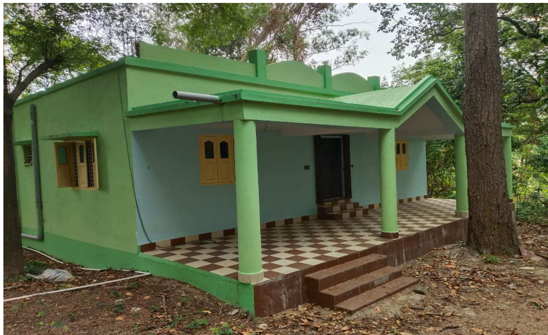
Construction of Dual Barrack at Arsha Beat under Purulia Division
