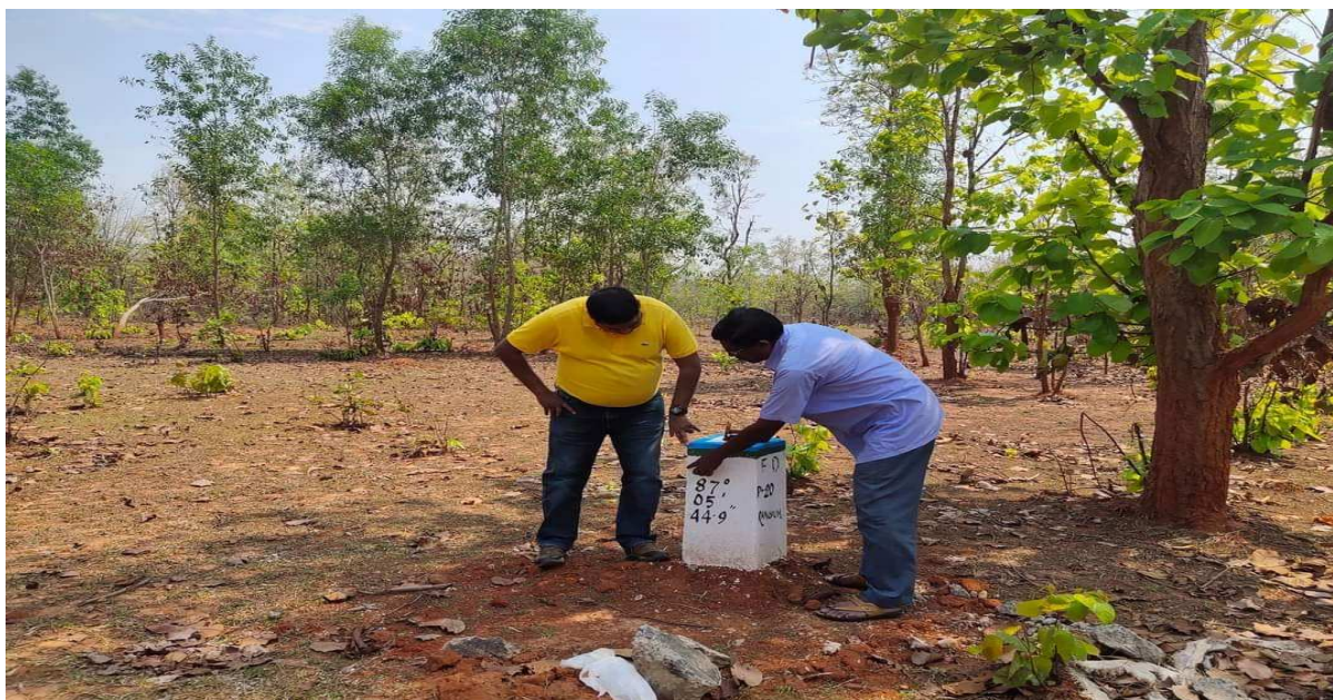
Erecting of Forest Boundary Pillar under Working Plan (South-I) Division
