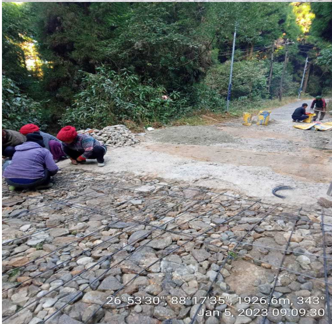
Construction of Causeway under Kurseong Range, Dowhill Beat, Dhobijhora Block Kurseong Division
