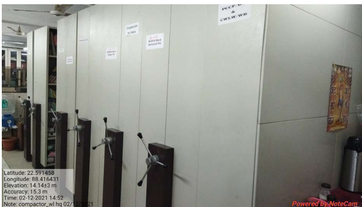
Wildlife HQ: Compactor
