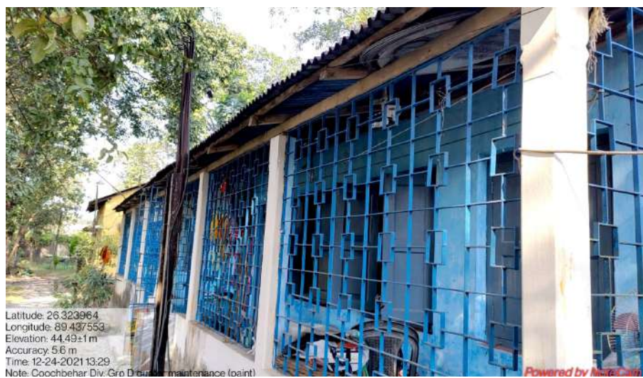
Cooch Behar Division: Maintenance of staff quarter
