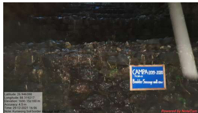
East Balason Catchment Range: Boulder sausage wall
