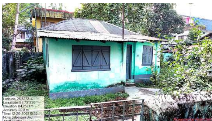
Jalpaiguri Division: Maintenance/renovation of staff quarter
