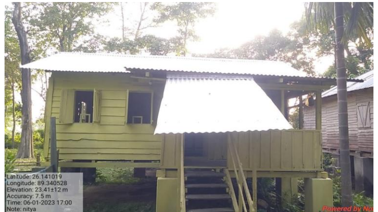
Repair of Group D staff quarter at Coochbehar Division
