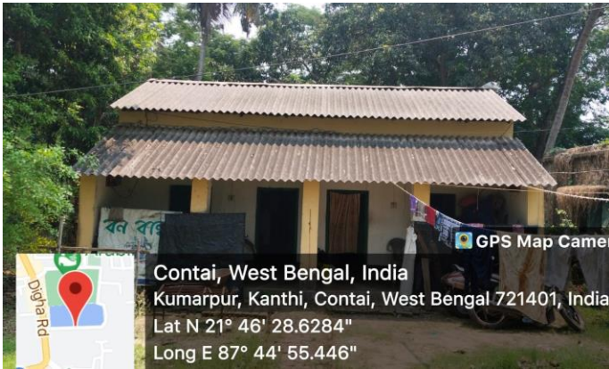
Repair of Group D staff quarter at Purba Medinipur Division
