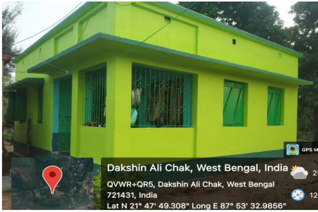
Repair of Group C staff quarter at Purba Medinipur Division
