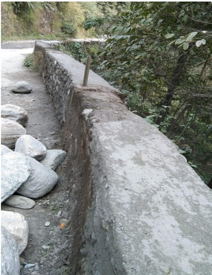
Construction of CRM Wall at Darjeeling Division
