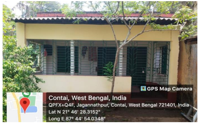
Repair of Group C staff quarter at Purba Medinipur Division
