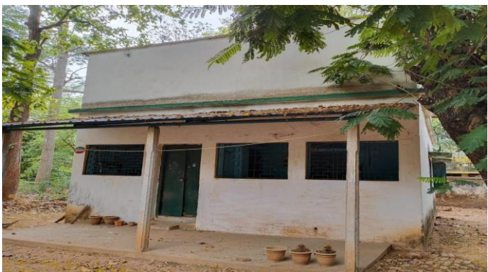
Repair of Group D staff quarter at Panchet Division
