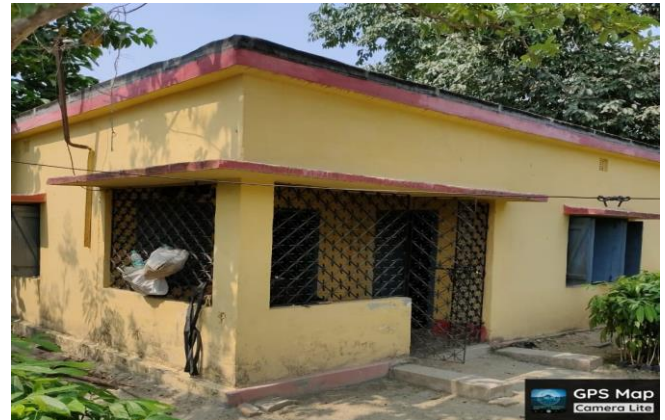
Repair of Group C staff quarter at Raiganj Division
