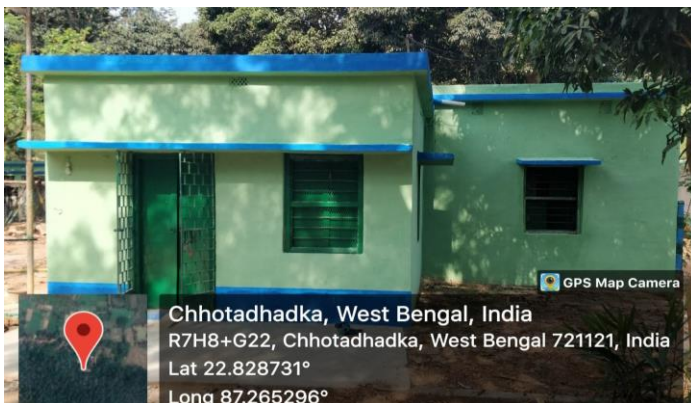
Repair of Group C staff quarter at Rupnarayan Division
