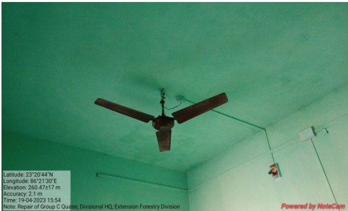
Repair of Group C staff quarter at Extension Forestry Division
