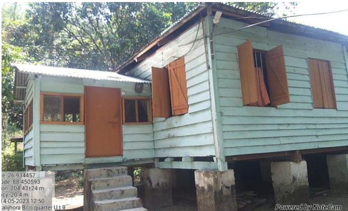
Repair of Group C staff quarter at Kurseong Soil Conservation Division
