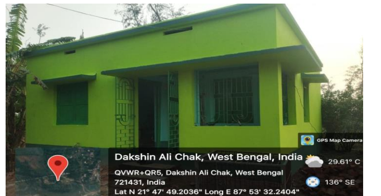
Repair of Group D staff quarter at Purba Medinipur Division
