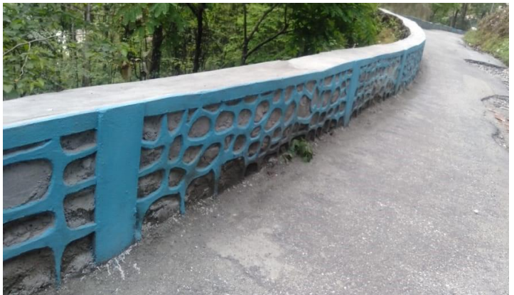
Construction of CRM Wall at Darjeeling Division
