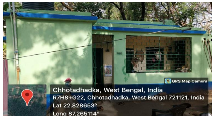
Repair of Group D staff quarter at Rupnarayan Division
