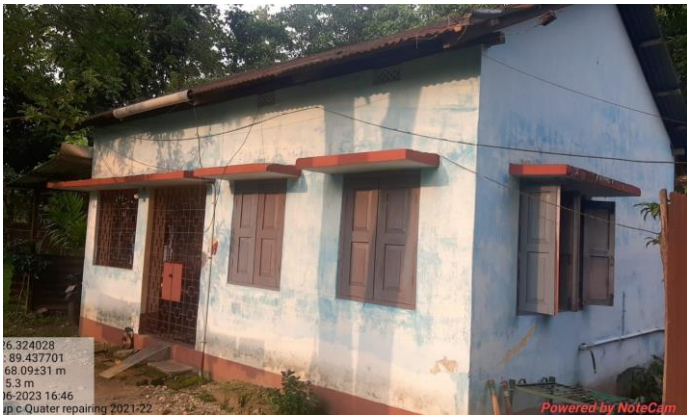
Repair of Group C staff quarter at Coochbehar Division
