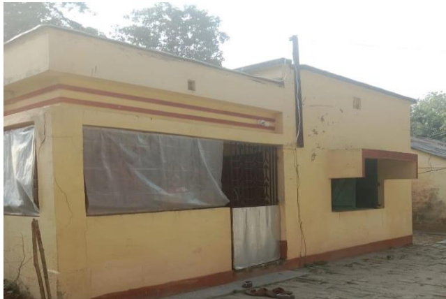
Repair of Group C staff quarter at Raiganj Division
