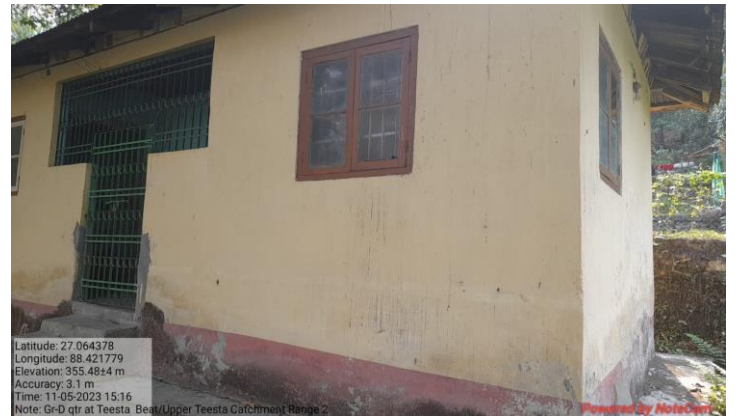
Repair of Group D staff quarter at Kurseong Soil Conservation Division
