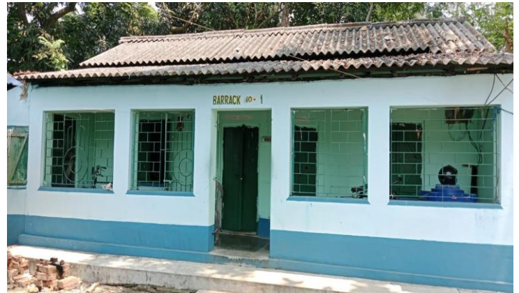
Repair of Group D staff quarter at Purba Medinipur Division
