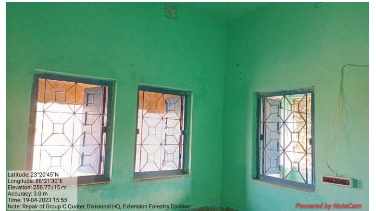
Repair of Group C staff quarter at Extension Forestry Division
