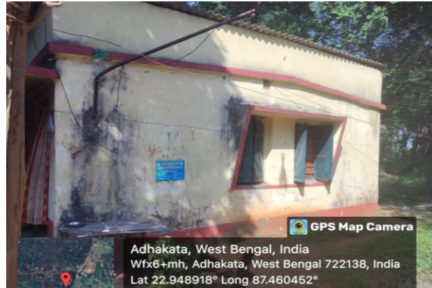
Repair of Group D staff quarter under Joypur Range, Panchet Division
