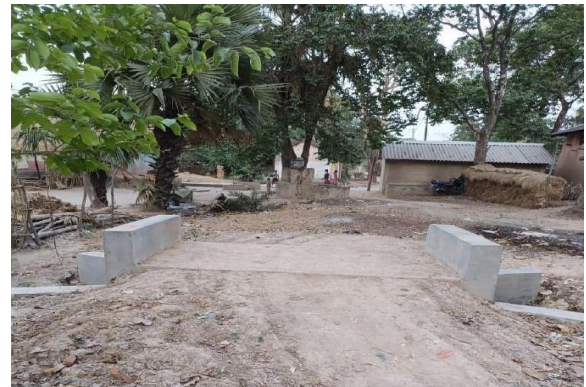
Construction of Culvert under Durgapur Range, Burdwan Division
