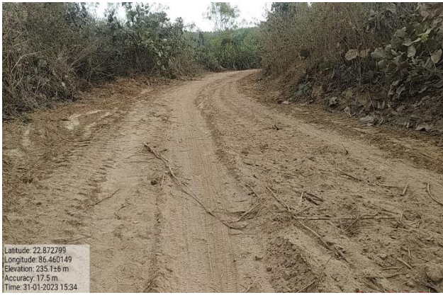
Repair of Forest Road under Bandwan I Range, Kangsabati South Division
