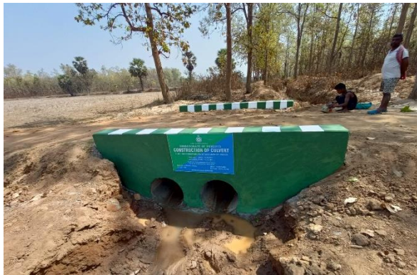
Construction of Culvert under Goaltore Range, Rupnarayan Division
