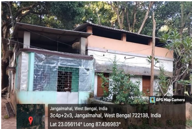
Repair of Group C staff quarter under Joypur Range, Panchet Division
